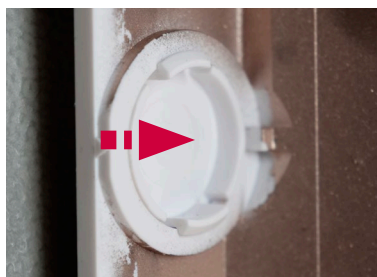
Figure 27 Install the cover if the VDI board has been removed
